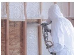
**PROS:** Has one of the highest R Value ratings of any insulating material out there. Closed cell foam insulation traps and
