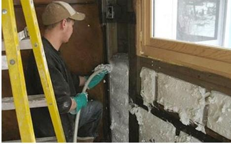
**PROS:** Very good sound insulation. No petro based chemicals used. Least toxic spray-in foam. Does not off gas. Fireproof. Doesn't shrink or settle. Mold resistant. No risk of blowing out walls during application. Not made of Portland cement but rather of magnesium oxide and magnesium chloride which requires 20%-40%
