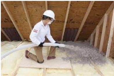
Cellulose insulation is created from a combination of wood and recycled paper. It works well when blown into existing wall cavities. In the application of new tiny house construction, only a wet, blown-in application makes sense.
